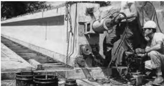
Figure I.25 – Post-Tensioning Jack Operating at an End of a Concrete Girder
